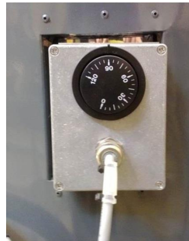
Figure 6 Flux heating control
